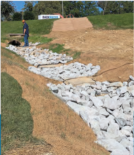
Clay Barber inspects a completed regenerative stormwater conveyance system.
