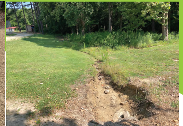
EDUCATIONAL OPPORTUNITY: (Above) An eroded swale on the Southern Nash High School campus; (left) the reconstructed swale runs with clear stormwater runoff. Courtesy of a Cummins Water Works grant, stormwater infrastructure is being built or repaired at public school campuses across Nash County. Assessments for 12 schools are currently underway.
