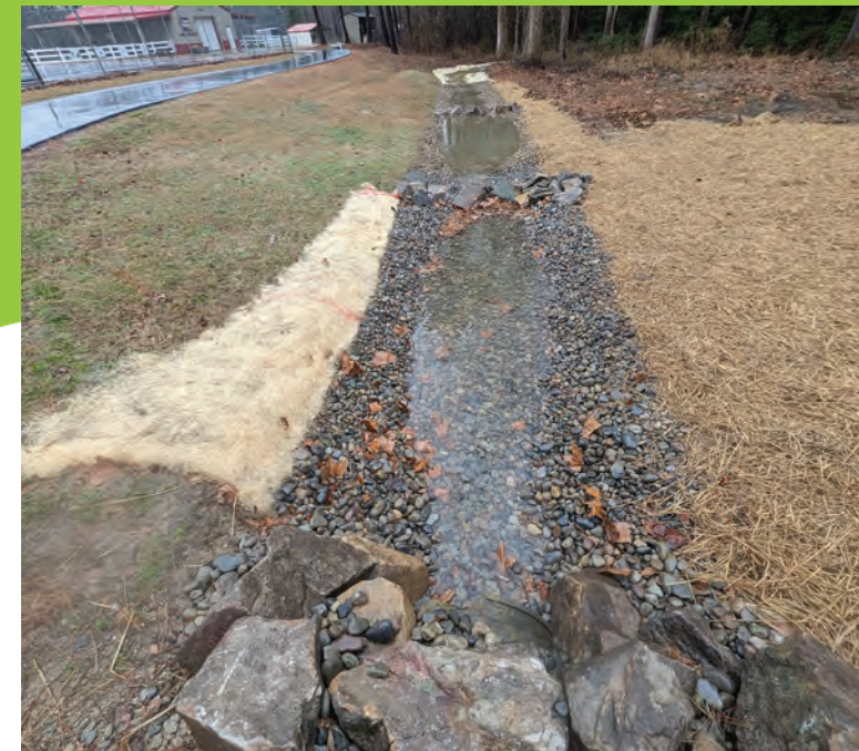
EDUCATIONAL OPPORTUNITY: (Above) An eroded swale on the Southern Nash High School campus; (left) the reconstructed swale runs with clear stormwater runoff. Courtesy of a Cummins Water Works grant, stormwater infrastructure is being built or repaired at public school campuses across Nash County. Assessments for 12 schools are currently underway.
