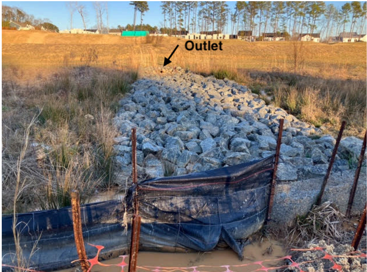
Attachment 1–Sediment filled runoff leaving a construction site near Ellerbe Creek headwaters
