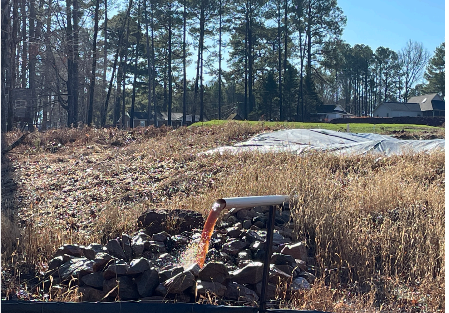
Attachment 4–Dirty discharge dewatering from sediment basin at edge of field, Lick Creek watershed (12/16/22)
