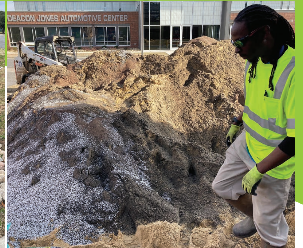
(Above left) The completed, restored bioswale is 1,700 linear feet of drainage for three acres of lawn and impervious surfaces at Wayne Community College. (Above right) Backwater Environmental Superintendent Chris Wheeler oversees the addition of the layer of soil, which was then topped by sod.
