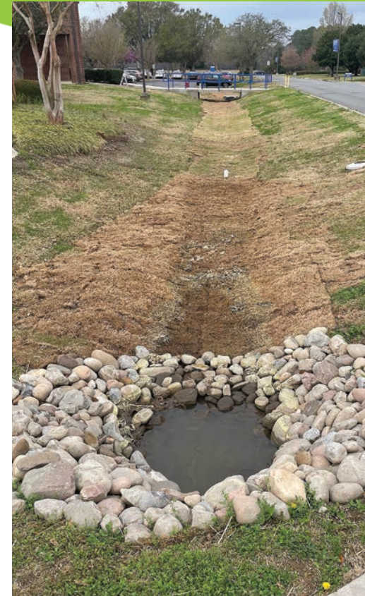
(Above left) The completed, restored bioswale is 1,700 linear feet of drainage for three acres of lawn and impervious surfaces at Wayne Community College. (Above right) Backwater Environmental Superintendent Chris Wheeler oversees the addition of the layer of soil, which was then topped by sod.
