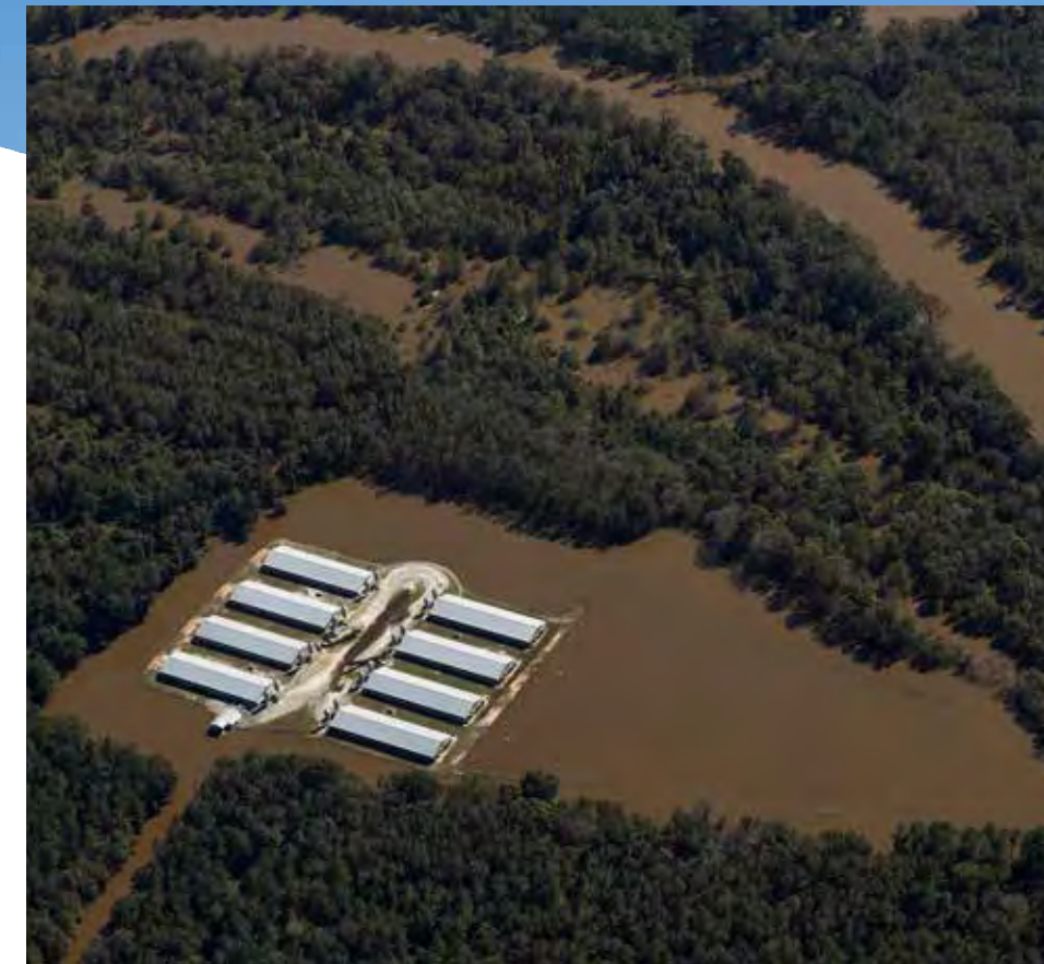
An industrial hog facility and inundated hog waste lagoon located in the Neuse watershed is pictured in the aftermath of Hurricane Matthew in 2016.
