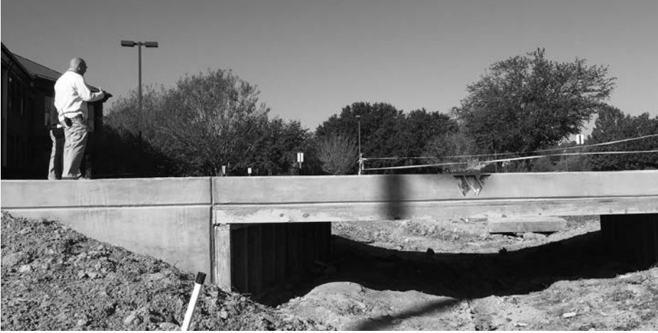
Derek Hunter, Wayne Community College vice president of operations, surveys an area where a Sound Rivers' stormwater project is planned.
