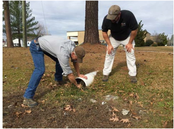
Mitch (NCSU) and Mr. Shaw (WCHS) examining drain pipe for cistern
