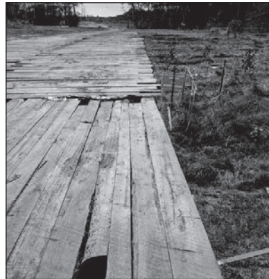
ACP construction route- Nash County near the Tar River in 2018
