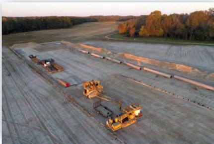
Contractors have drilled under the Tar River, cleared land and staged pipe on both banks of the river in Nash County (Left)
