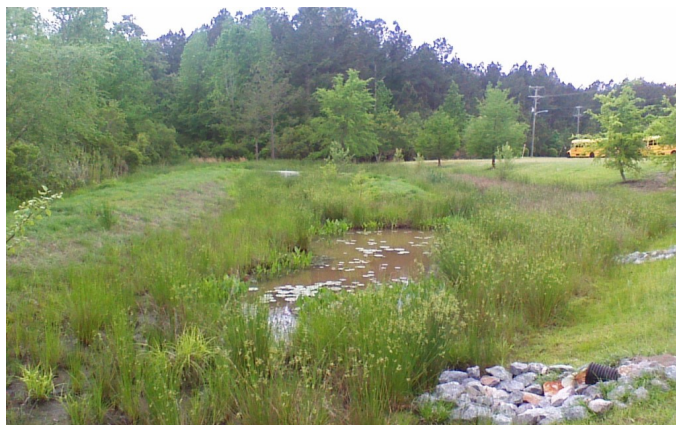
Created wetland two years after construction.
