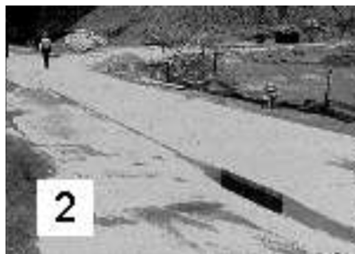
Figure 2. Proper establishment techniques can prevent soil erosion.
